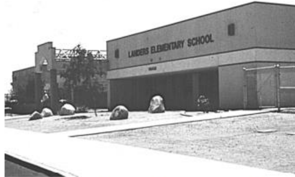
Figure 4 Landers Elementary School with minor non-structural damage and immediate reuse after the 7.3 magnitude 1992 Landers earthquake. There has been no partial or full collapse of any public school building constructed to the requirements of the Field Act since 1933.
